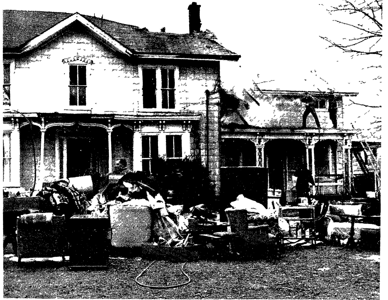
Two Family Home in Salem Guttled by Fire Last Week Wednesday
