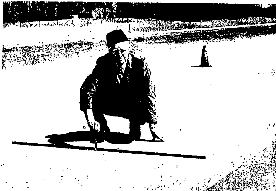
COBBLESTONE—State Representative James Tierney, chairman of the House Public Safety Committee, demonstrates on I-696 the cobblestone street-type surfacing beginning to appear on many Michigan highways. The culprit, he and others maintain, is metal-studded tires.
