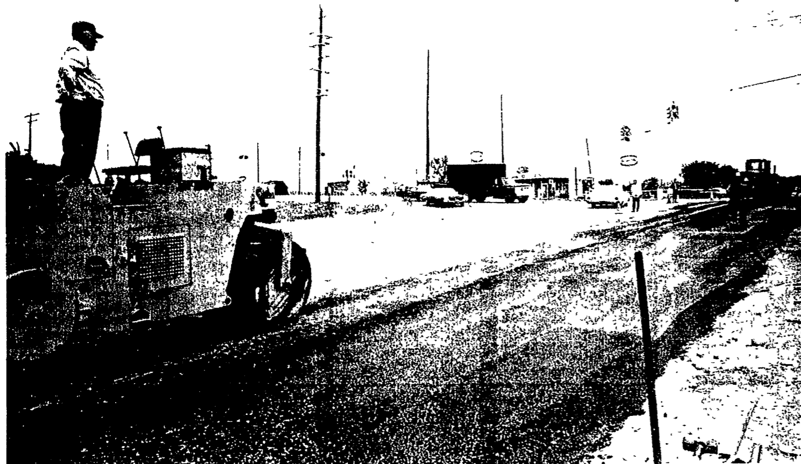
EXTRA LANE—Wayne County Road Department workmen began construction of an extra south-bound lane on Northville Road at Seven Mile last week. When completed
