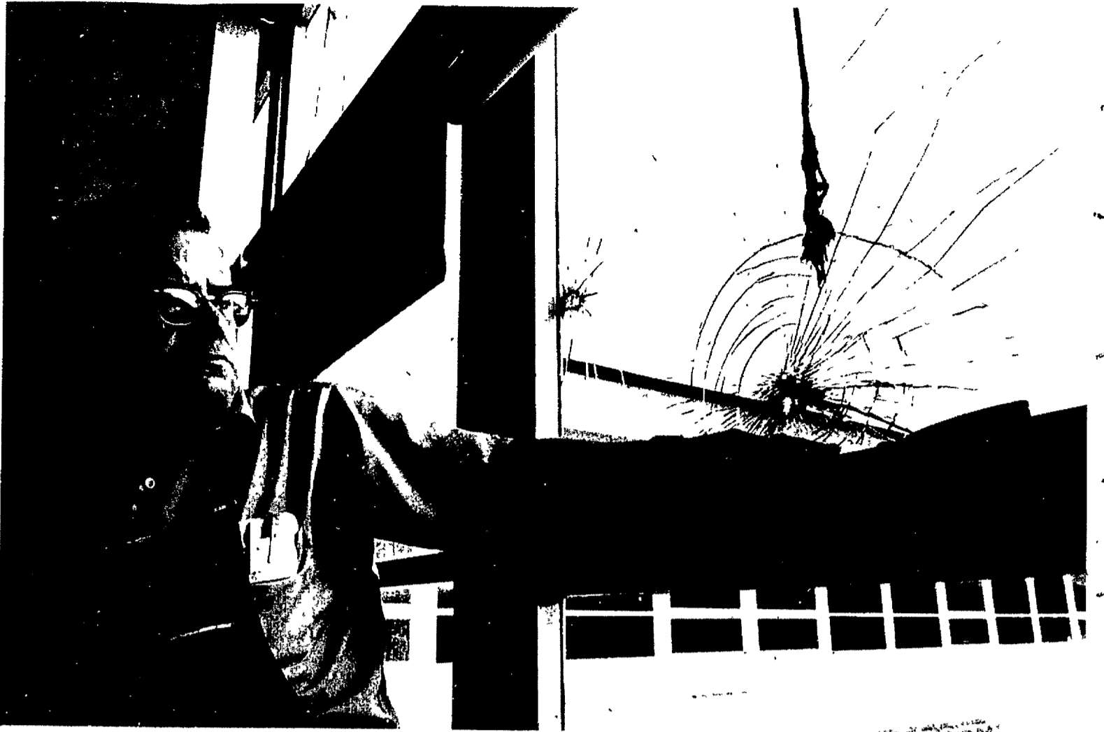
IT HURTS—Vandalism is a regular nemesis of area school systems, hurting both the pocketbook and the districts' pride. Elementary School in South Lyon, inspects one of 31 damaged windows at the school. Above, Dallis Richardson, building engineer at Sayre
