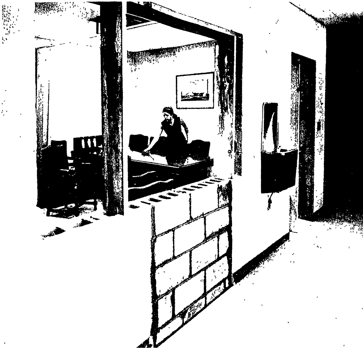
NEW OFFICE —Moving of a door and provision for windows signalled the start of remodeling this past week of the council conference room, which is to serve as a clerk's office in the city
