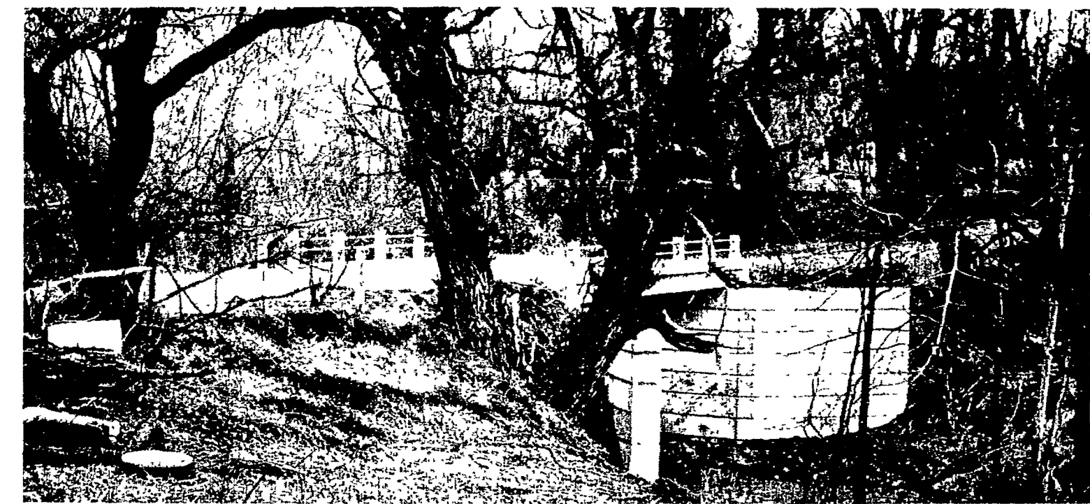
IT'S OPEN — Although work on the approaches, storm drain, and cleanup remains to be done, the new bridge over the stream on the Rural Hill Cemetery Drive has opened for traffic. The concrete structure replaces the old, often-
