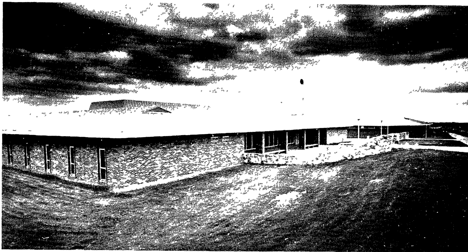
Trustees toured the new Applied Science addition at nearby Schoolcraft College officially signalling its completion
