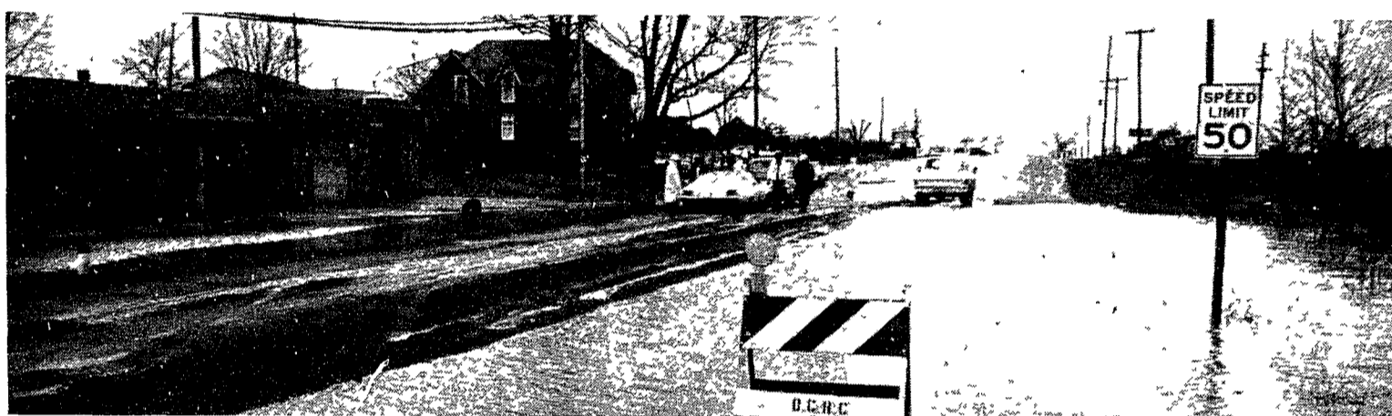
A Blocked Storm sewer Created a Traffic Hazard by Covering Grand River Avenue with More than Two Feet of Water
