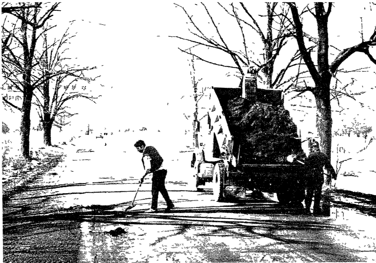
County workmen patch pre-spring chuckholes in Eight Mile Road
