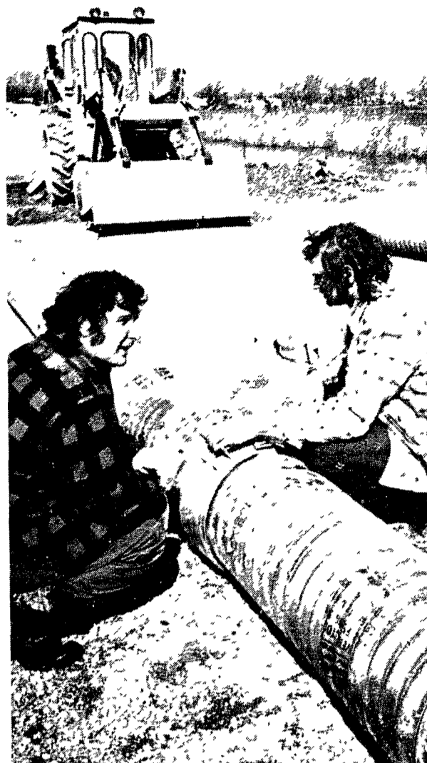
Workmen Install Additional Drainage Pipes
