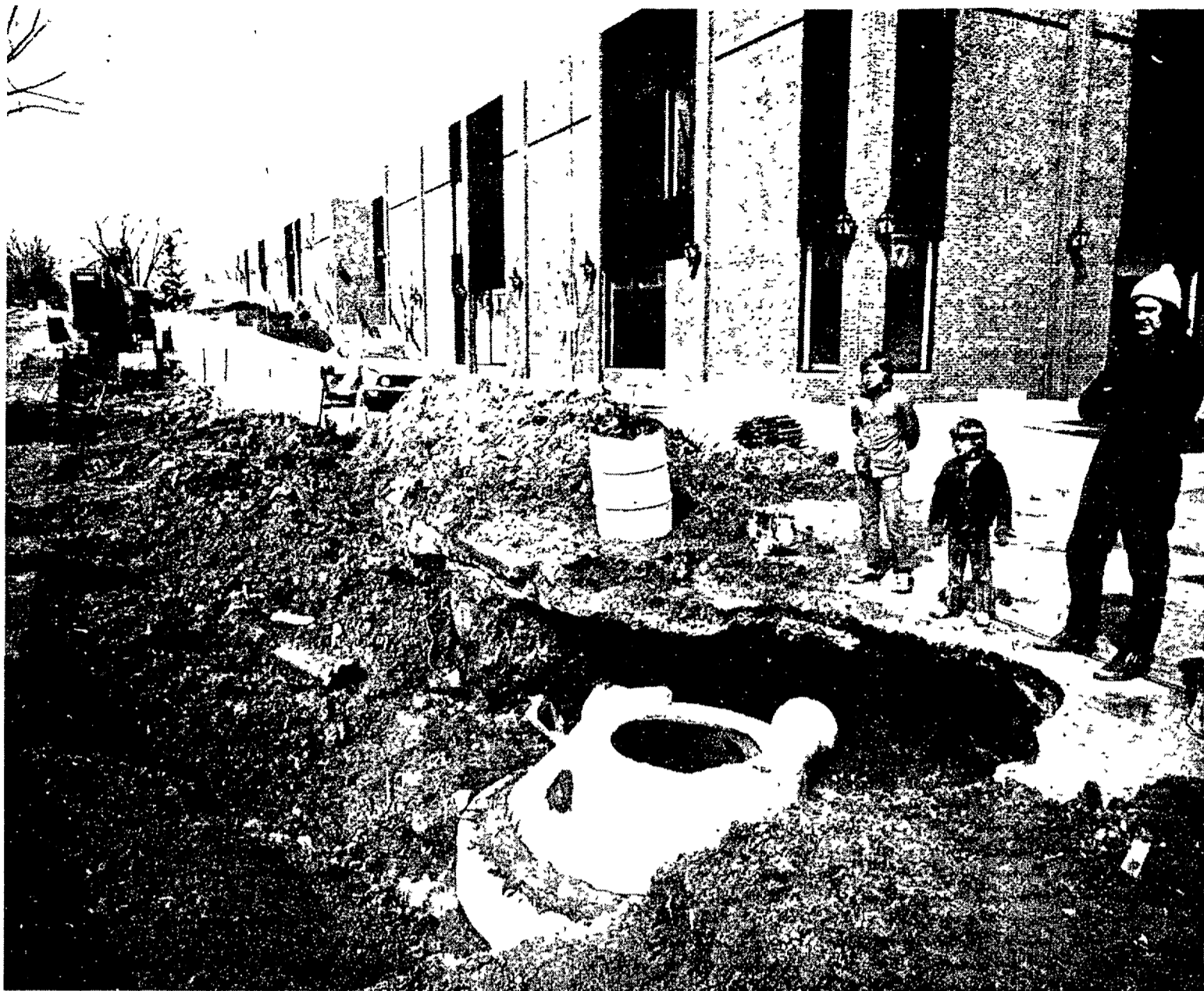
BLOCKED —Installation of water and sewer lines began this past week on Wing Street, between Cady and Main, forcing motoring detours to and from and post office.
