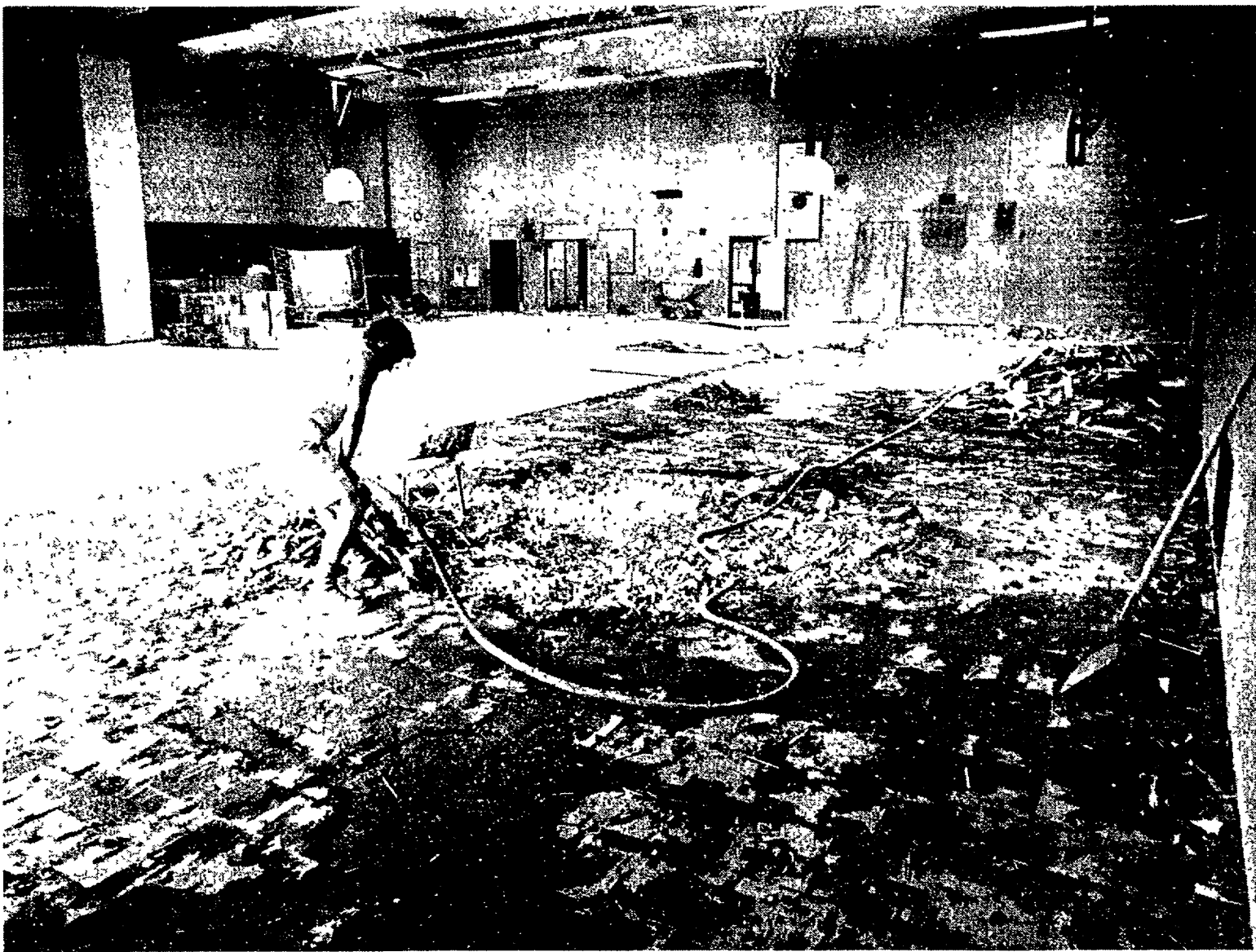
GYM EXCAVATION — Cooke Middle School's gymnasium floor is undergoing repairs as workmen dig out the fill beneath part of the floor. The work, a result of the out of court settlement with the contractor and architect of the school, is expected to be completed by September 15. Fill
