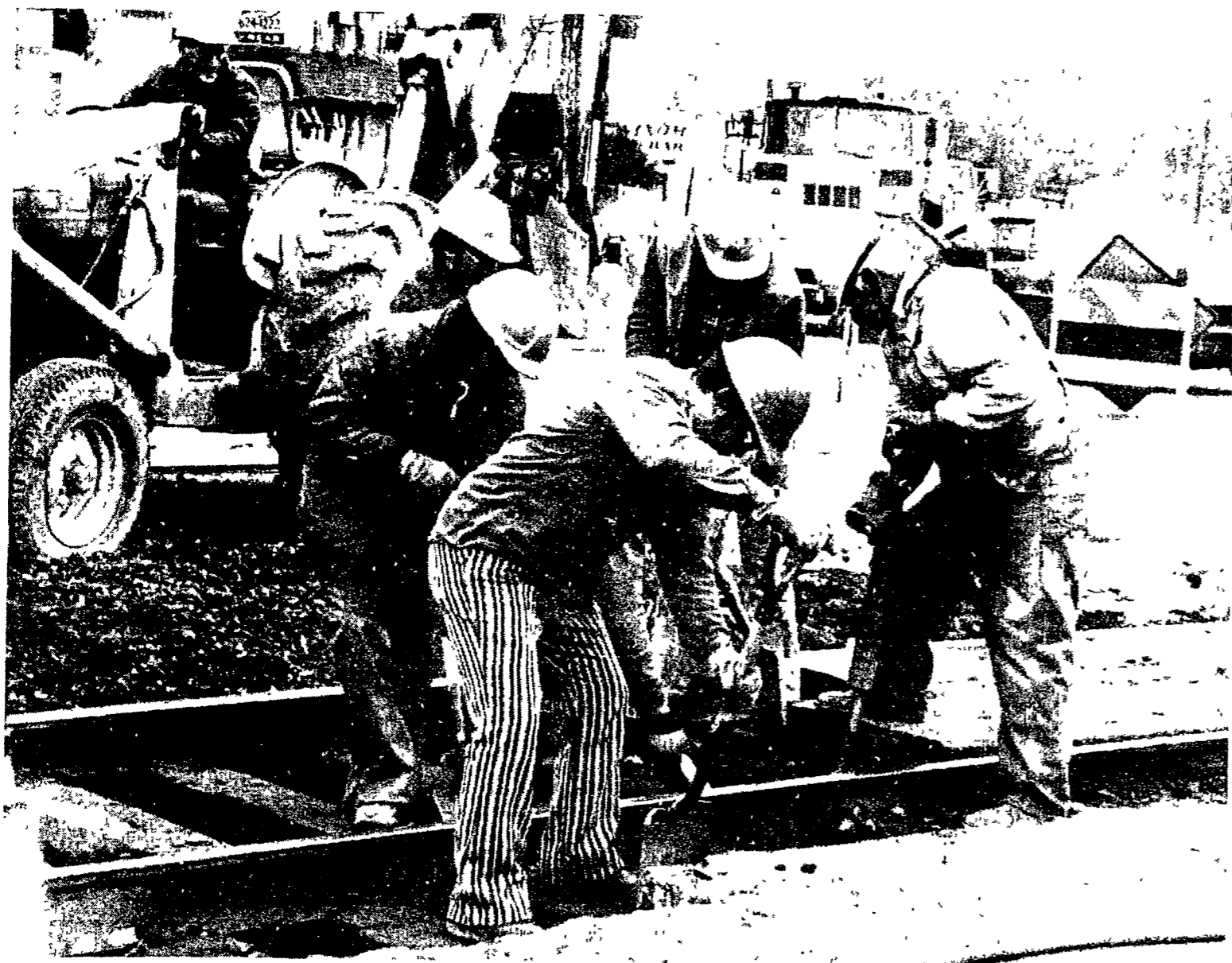
WORKING ON THE RAILROAD —Workmen from the Chesapeake and Ohio Railroad tear up the Wixom crossing at Pontiac Trail and Wixom Roads. The intersection in Wixom has been a constant source of complaint because of
