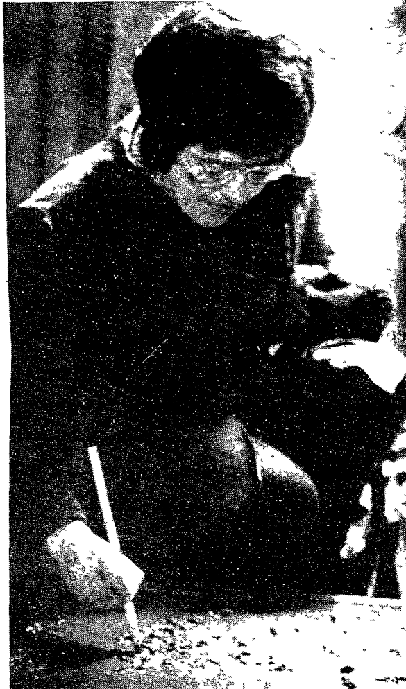
LASTING MEMORY —Novi City Clerk Gerry Stipp draws her name in wet concrete — one of dozens of officials and citizens who did so following the groundbreaking ceremony for the new Novi High School at the corner of 10 Mile and Taft roads. The "memory slab" is to be displayed somewhere on the high school property when the new facility is completed.
