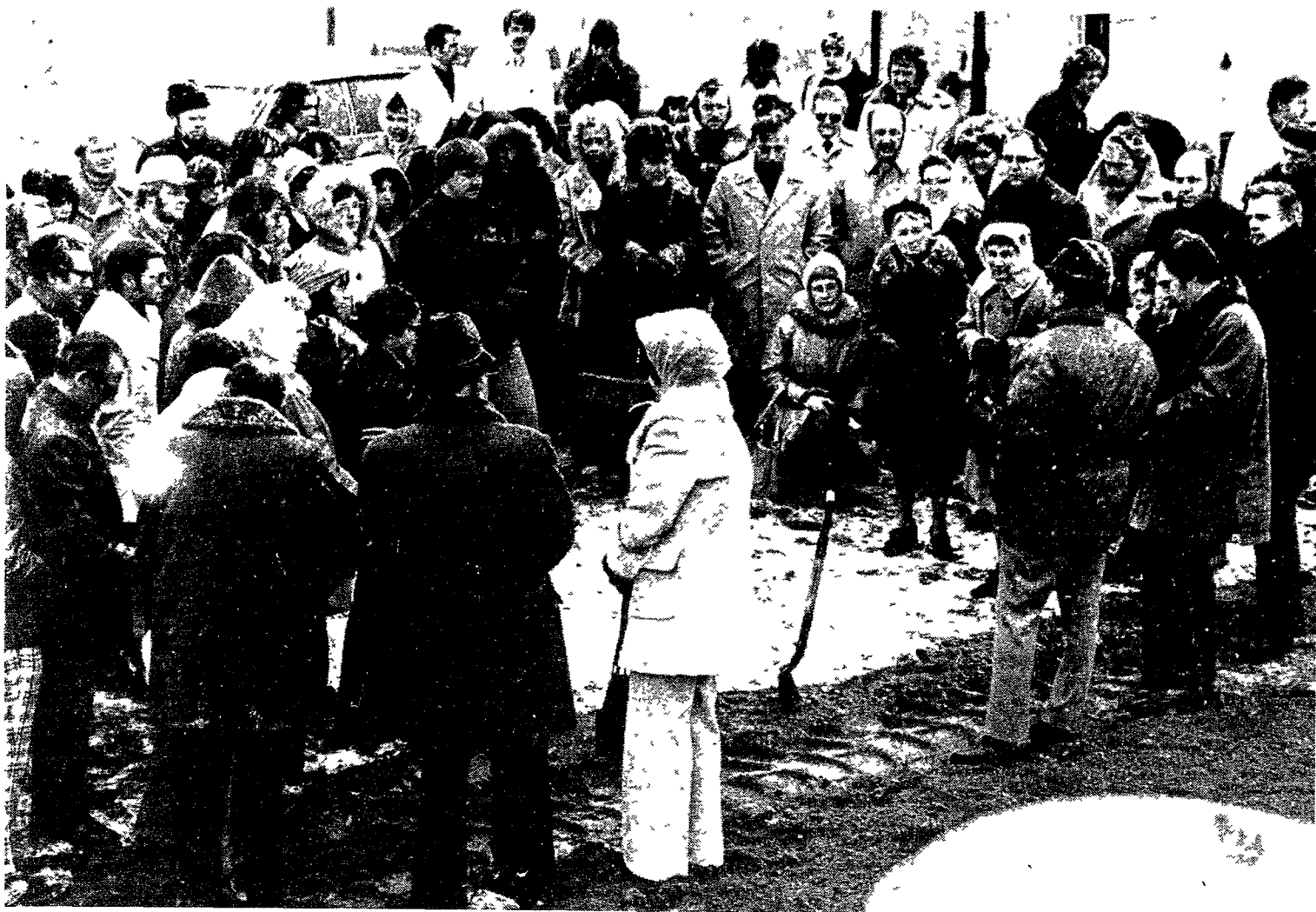
GROUND BREAKING —Despite snow flurries and cold weather, groundbreaking ceremonies for the new Novi High School came off without a hitch last week Wednesday. Here, grouped in a circle listening to some words from School Board President Robert Wilkins (back to camera, bottom right), are some of those who attended. Standing next to him (right) is Father Leslie Harding who offered
