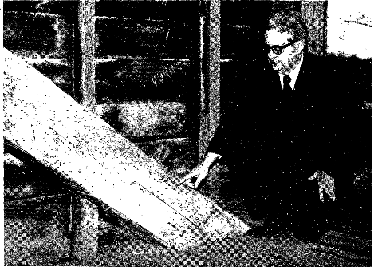
NORTHVILLE RESIDENT Blake Couse points to a repaired timber in Greenfield Village's Ackley Bridge. Repair work by his
