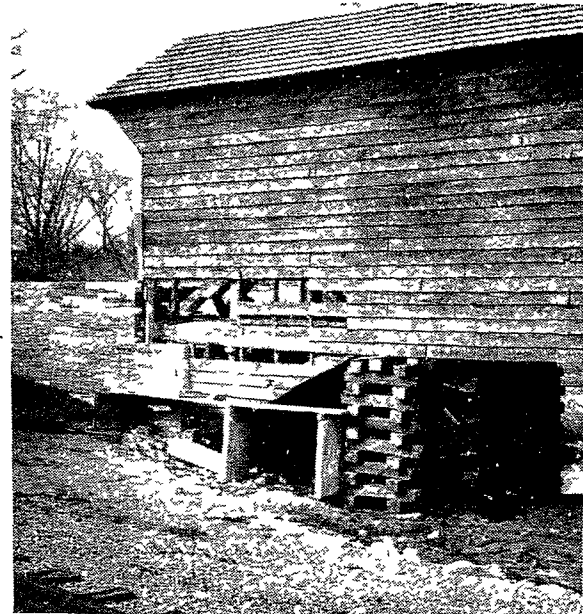
Covered bridge braced for construction work
