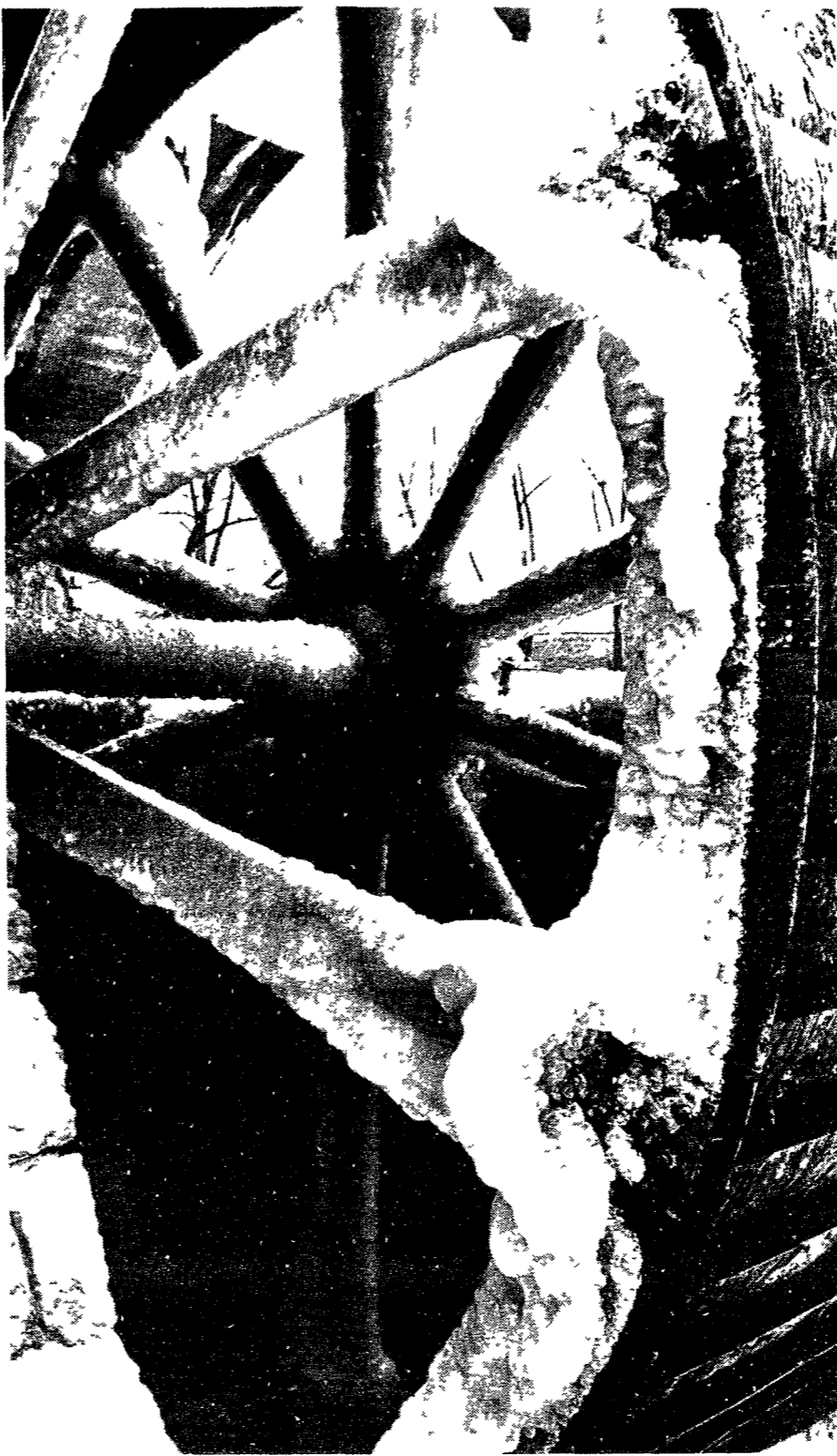
Ford Valve Plant water wheel takes a winter rest beneath blanket of ice
