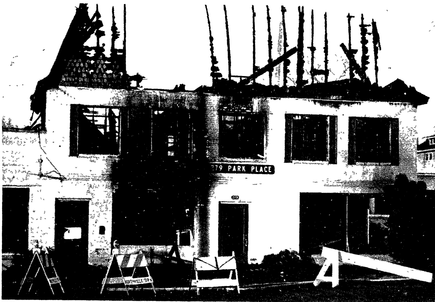
Not much more than the four walls remain of this old Northville building following the fire Monday morning
