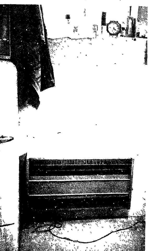
ELECTRIC HEATERS —The tack rooms throughout Northville Downs are serviced by electric heaters to lessen the chance of an explosion and a resulting fire.
