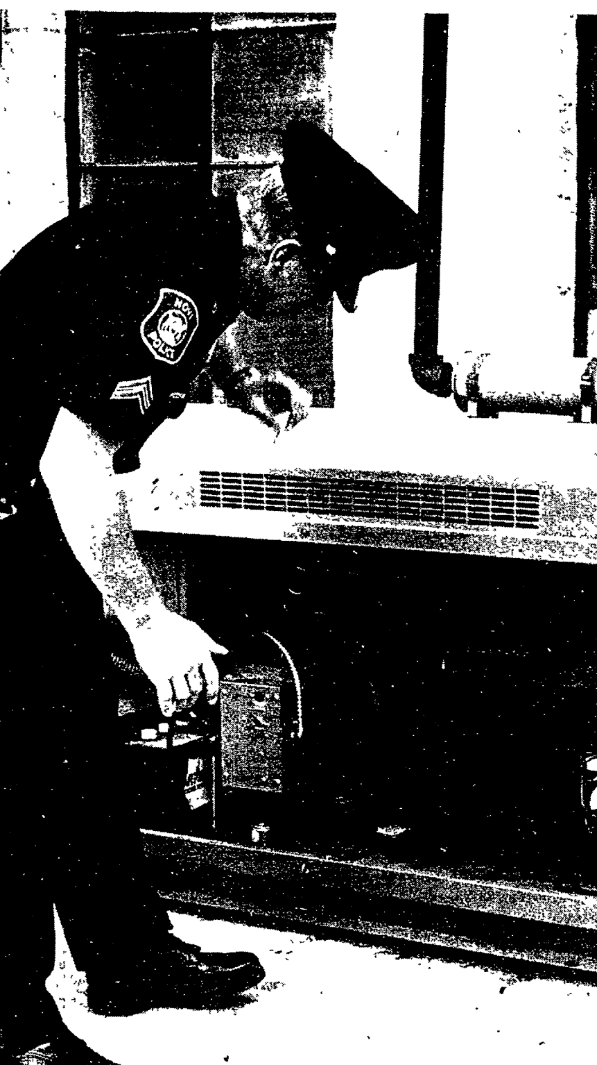
NEW GENERATOR —Corporal Ralph Fluhart of the Novi Police Department looks over the new police generator recently put into service. The generator, which runs on gasoline, starts automatically in an emergency if power is disrupted at the police station. The generator will enable the department to continue using the teletype machine, police and fire monitors, telephones and lights.
