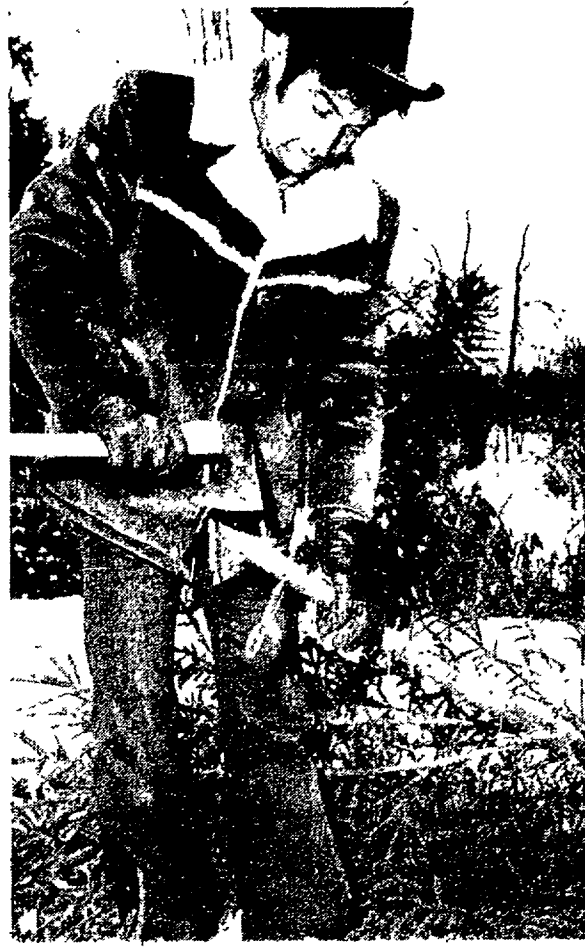
SHARPEN the top of the tree trunk so you can pound it into the ground.
