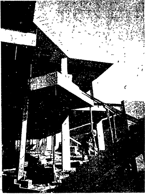
Novi's new high school got underway at 10 and Taft
