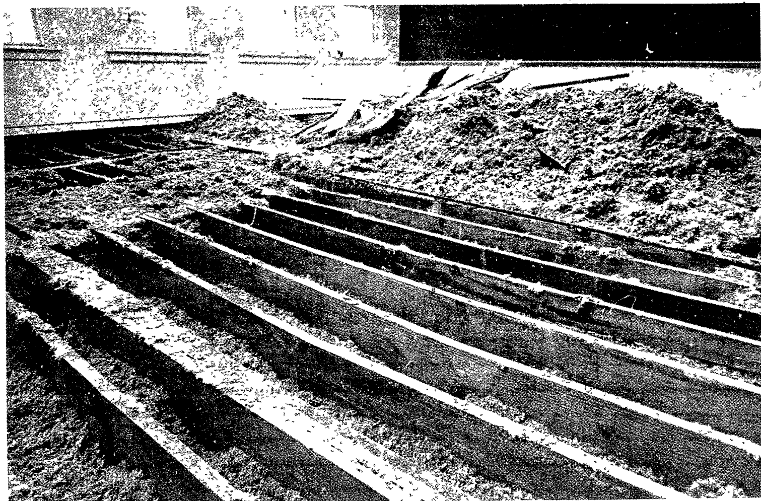
Six of nine exposed beams revealed cracks
