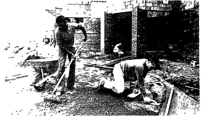
New township hall complex got underway
