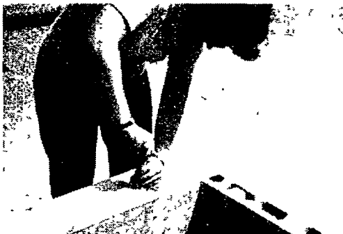
Screws pin the sill to wooden blocks
