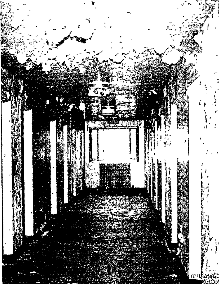
A malfunctioning of the steam heating system caused this damage
