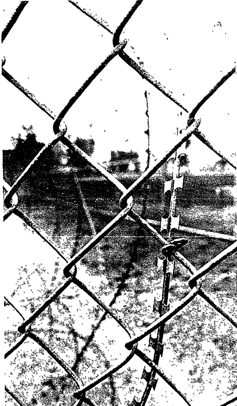
Razor-sharp concertina wire adds to chain link fence security
