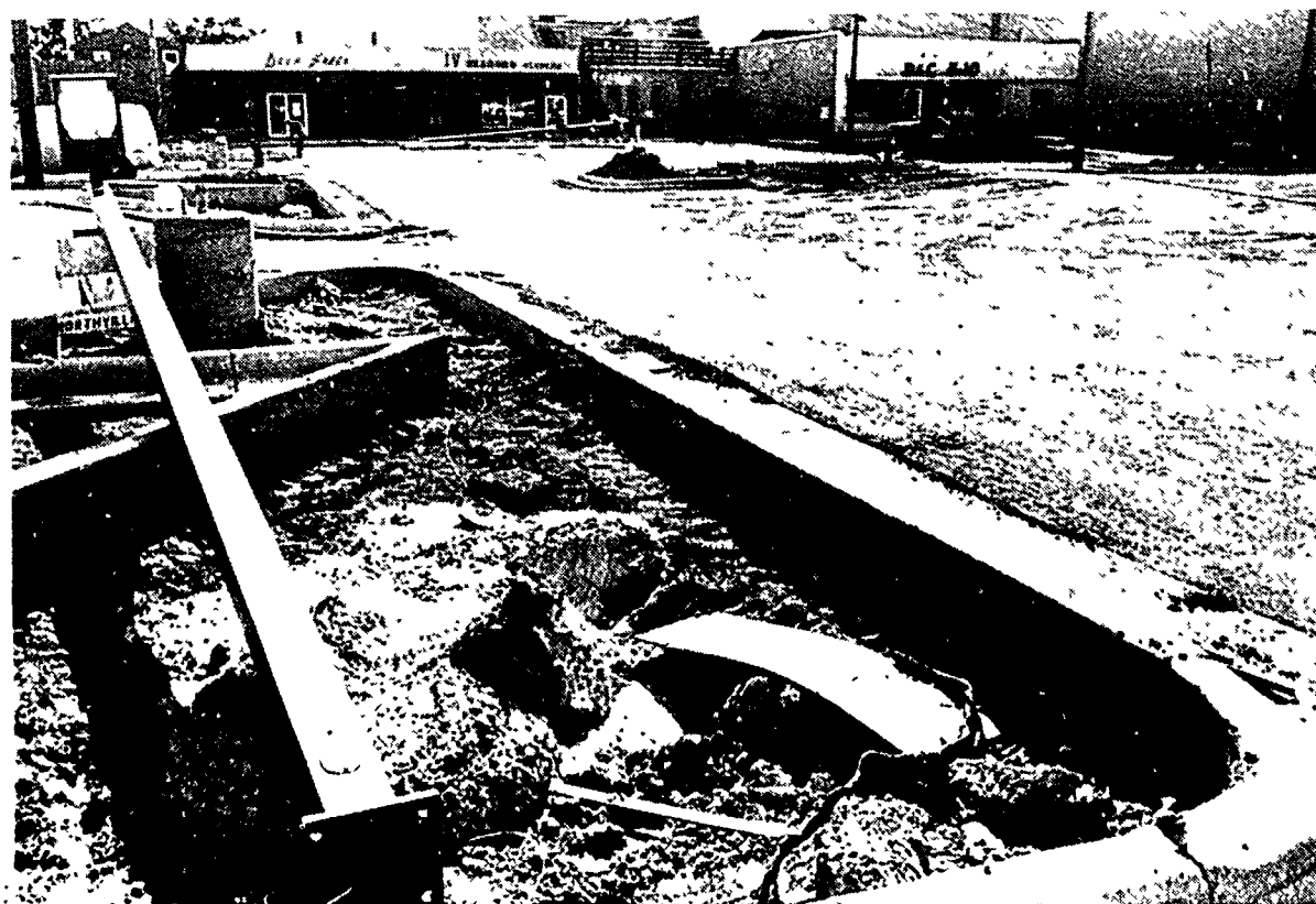
Curbing's in with paving to be finished this week
