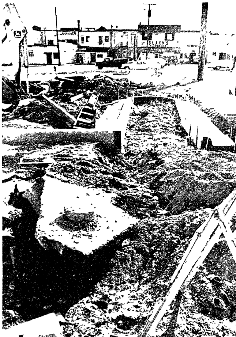
Grading provides a smooth sweep of parking lot to Dunlap Street
