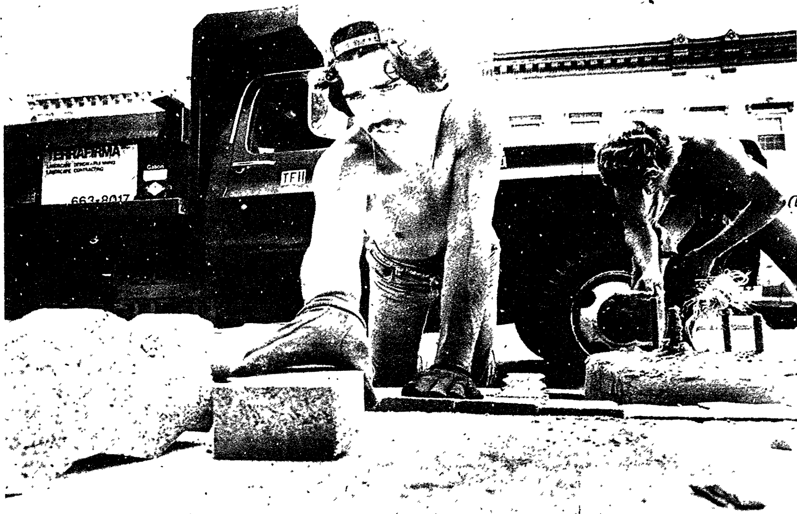
BRICKLAYING — Matt McClear and Tim Powell, background, lay bricks in the sidewalk as part of the Main Street project
