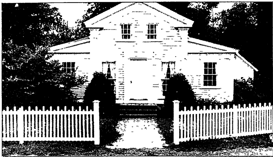
New fencing encloses Hunter House garden
