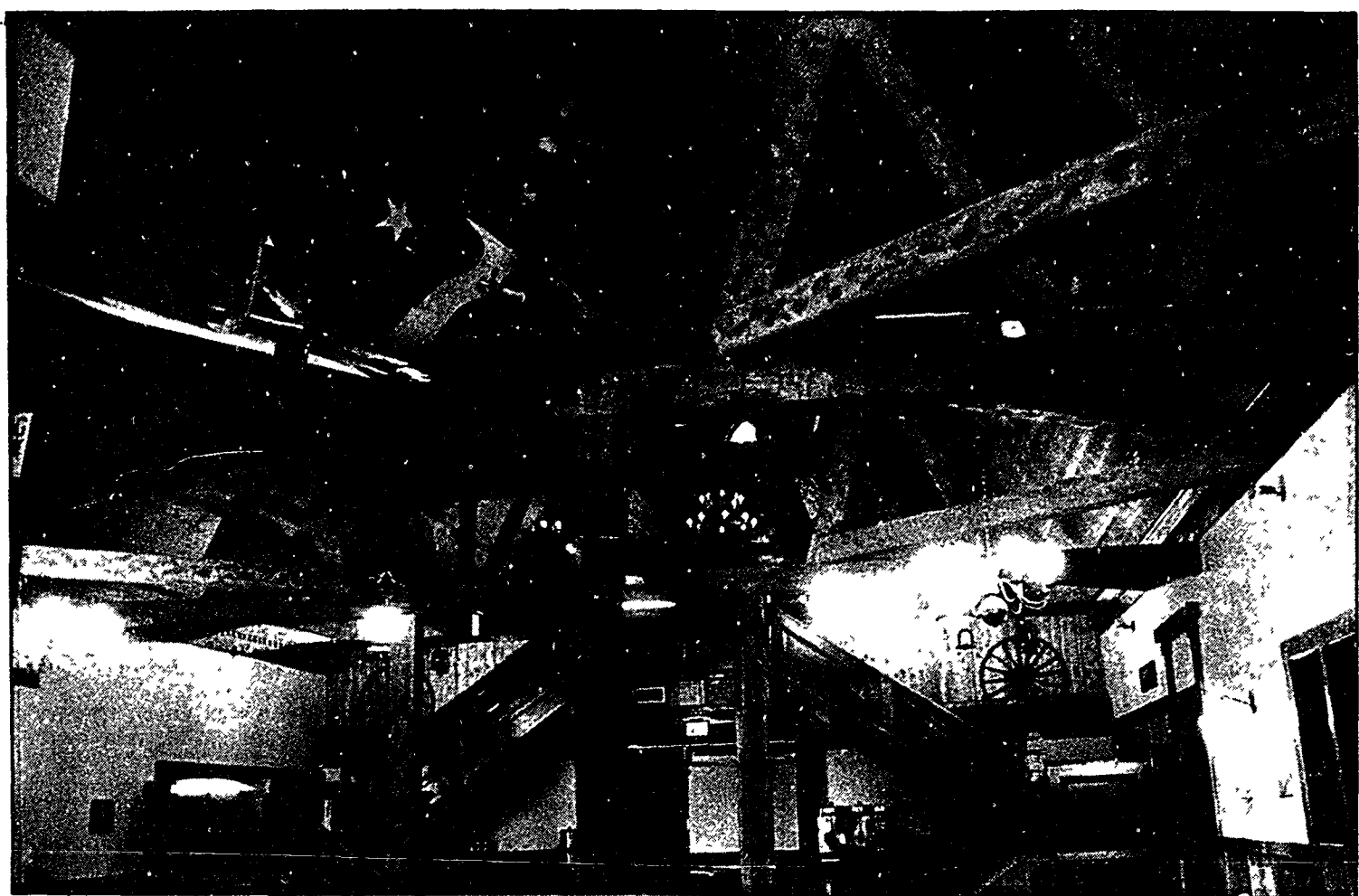
Double scissor beam roof construction gives Barnstormer restaurant room to hang a plane above diners
