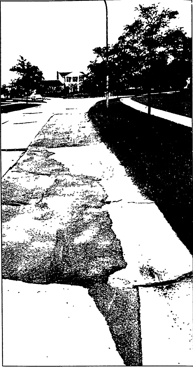
Fairfax Court pavement buckled due to erosion of subsurface
