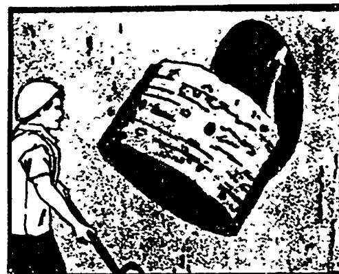
30" HOLE DRILLED 2 FT. DEEP IN HEAVILY REINFORCED CONCRETE.
