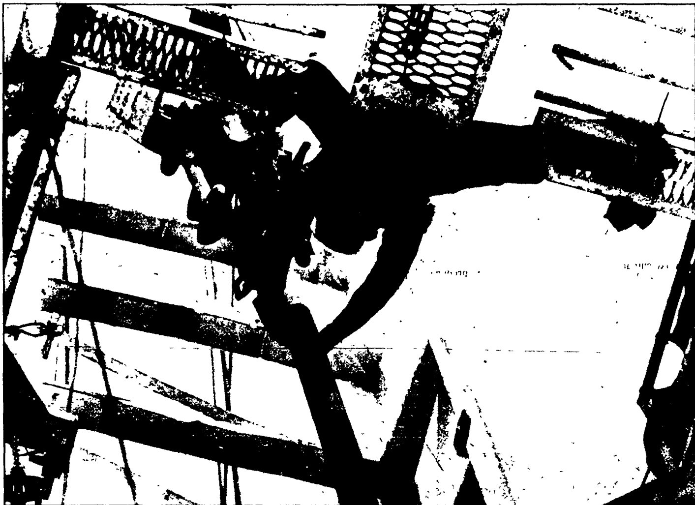
Derrick man Mike Lapham steadies drill pipe 50 feet above the drilling floor
