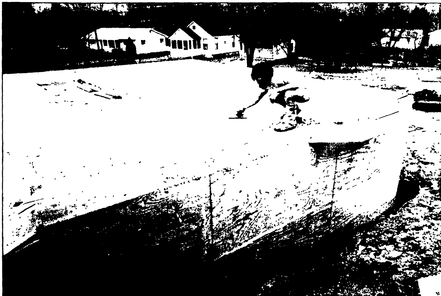
Bill Gourlay smooths out the cement floor built atop a wooden foundation in an Integral Works home.
