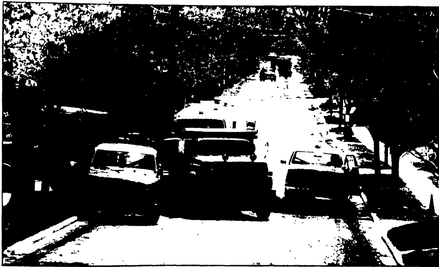
Road work begins
