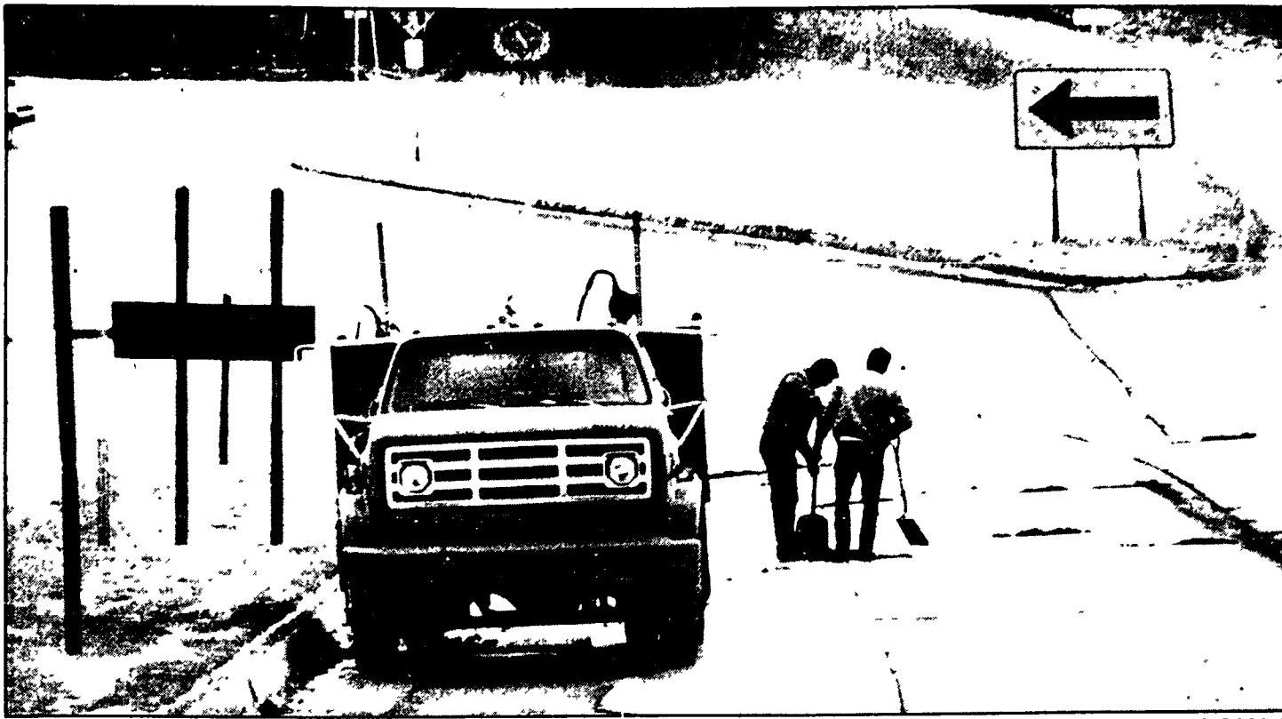
The Oakland County Road Commission was out repairing potholes recently, at Eight Mile near Taft Road.
