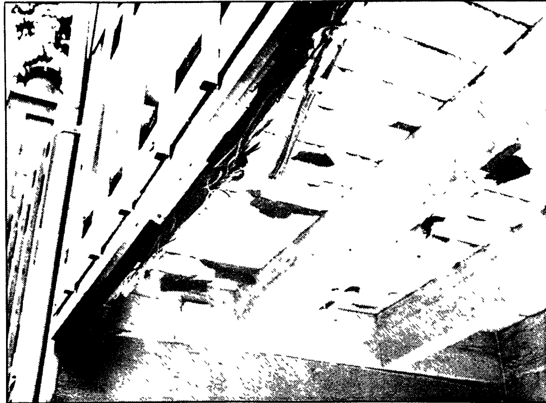
Rotting support beams on a balcony at Innsbrook Apartments.
