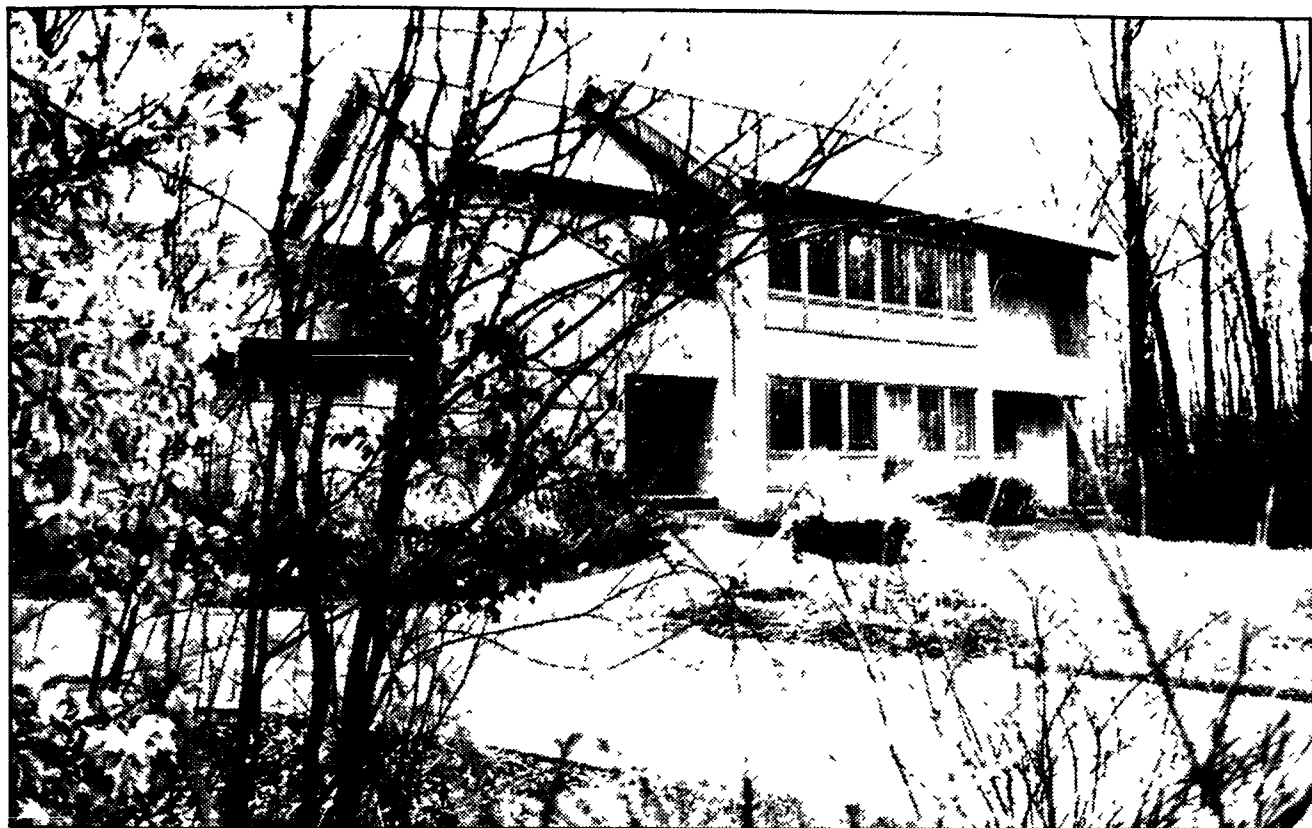
Saving trees and maintaining a natural setting was a priority for the Coxes when building their new home in Novi.
