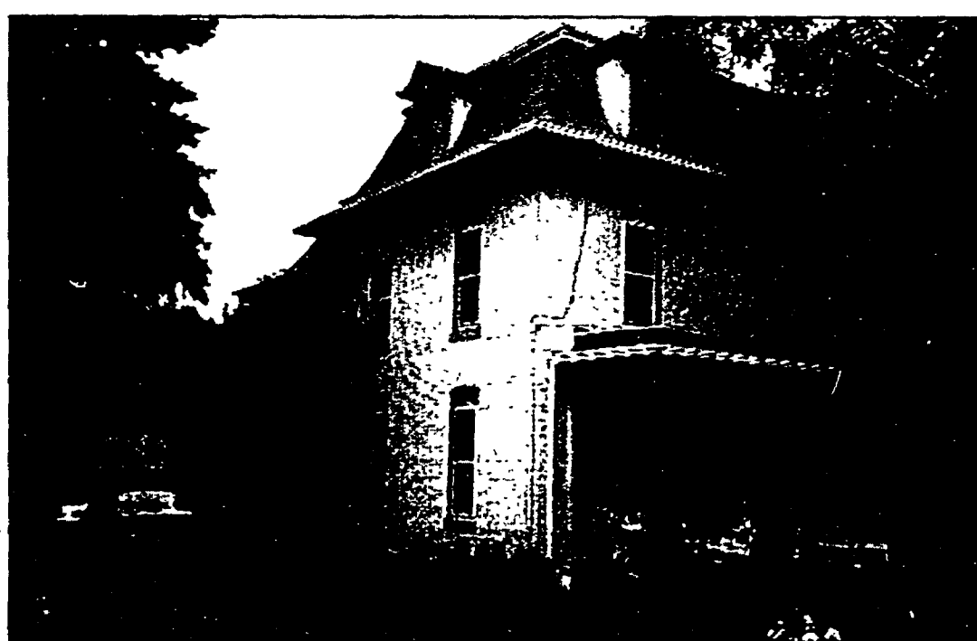
The Mansard roof allows the third floor or attic of this home to be used as living space.
