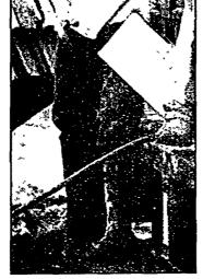
Above: Rougher Clinton Williams, balancing on the partition wall of a home under construction, works on nailing together support beams.
