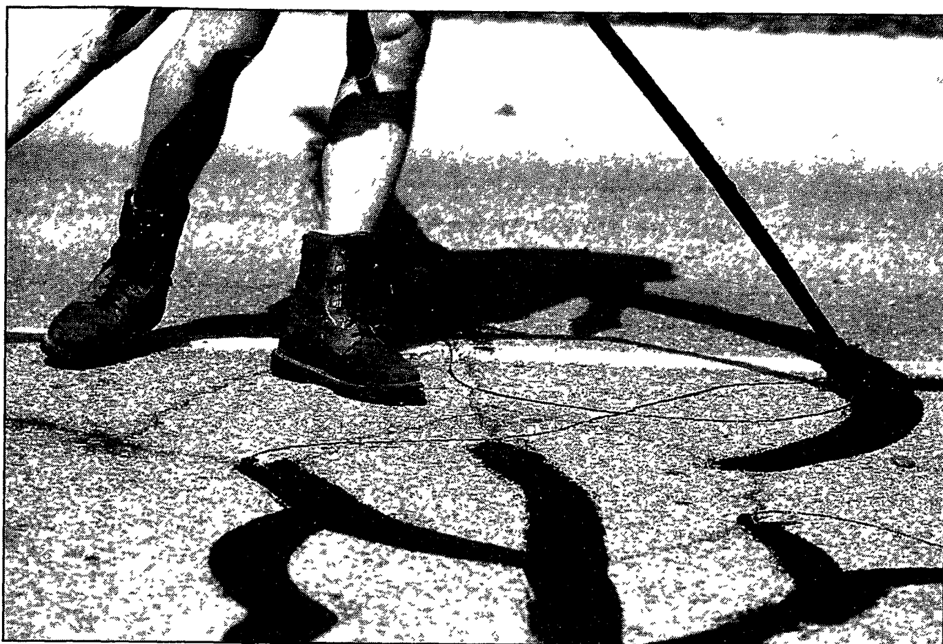
Crew members like Marc Tolsdorf go through one pair of work boots each summer because of the intense heat of both the torch and applicator used in the hot patch road repair. Right: Bob West uses the torch to remove old tar, debris, and moisture from cracks that have formed in the road surface.
