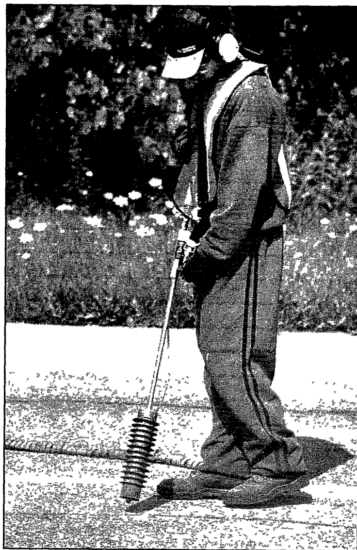
Crew members like Marc Tolsdorf go through one pair of work boots each summer because of the intense heat of both the torch and applicator used in the hot patch road repair. Right: Bob West uses the torch to remove old tar, debris, and moisture from cracks that have formed in the road surface.
