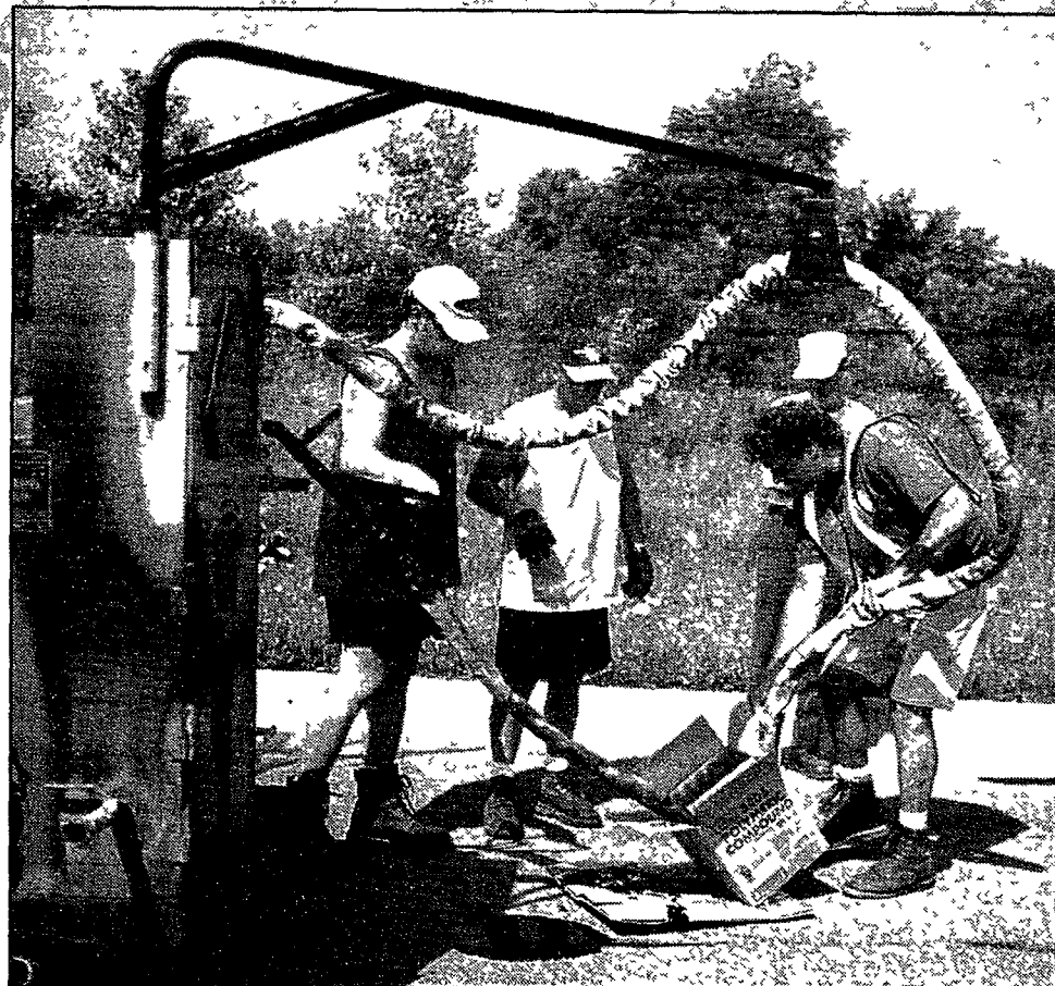
Crew leader Tim Wright, right, puts the hot tar applicator hose into a box to contain the spill caused by the hose springing a leak, that stalled the patching efforts for morning.
