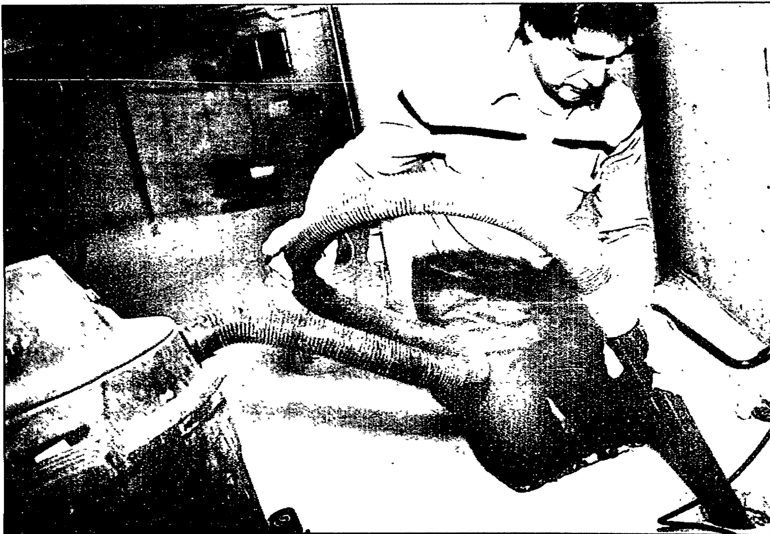
Earl Wall of Radon Management Systems cleans the area where he's building a pipe system that will take radon gas from the ground beneath this home and release it through the roof. Radon, a naturally produced gas, is a health hazard. Long-term exposure to the gas causes lung cancer.
