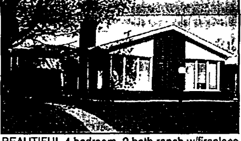
BEAUTIFUL 4 bedroom, 2 bath ranch w/fireplace in living room. Fantastic finished basement. With dry bar, work out room. Newer windows. 2 1/2 car garage w/fenced yard. (89INK) $154,900. 734-455-5600.
