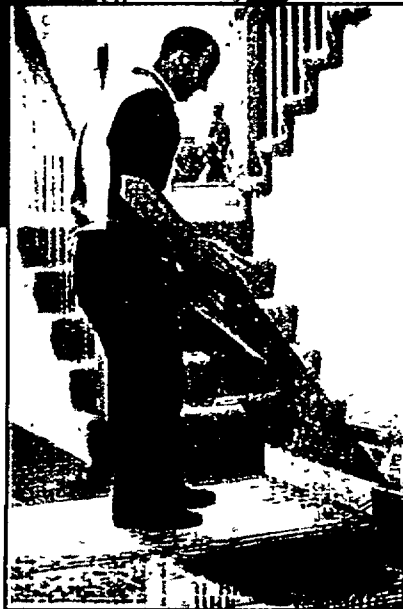
Top: Greg Young of Solar Shield in Novi, applies a film that reduces 99% of the sun's UV rays that cause fading in carpet and furniture. Above: The Solar Guard film is sized and cut on site for a perfect fit.
