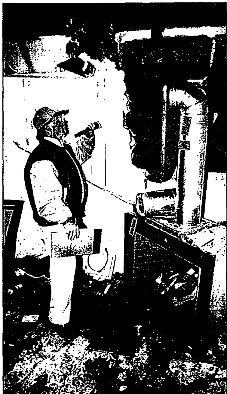
Northville city building inspector Rick Starling, left, takes a look at what can happen when city codes are not followed: a fire broke out last week in this Northville home off Grassmere after a fireplace flue was improperly installed. More than a third of
