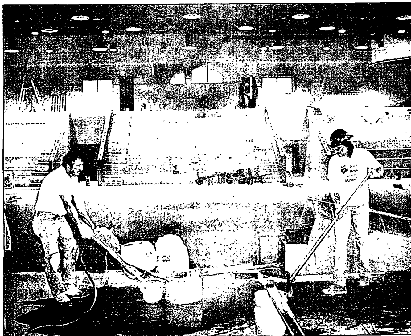
Concrete floor finishers Tom Rotodi, left, and Dave Thompson work on smoothing out the partially finished theatre stage floor at the new Northville High School last Thursday morning.
