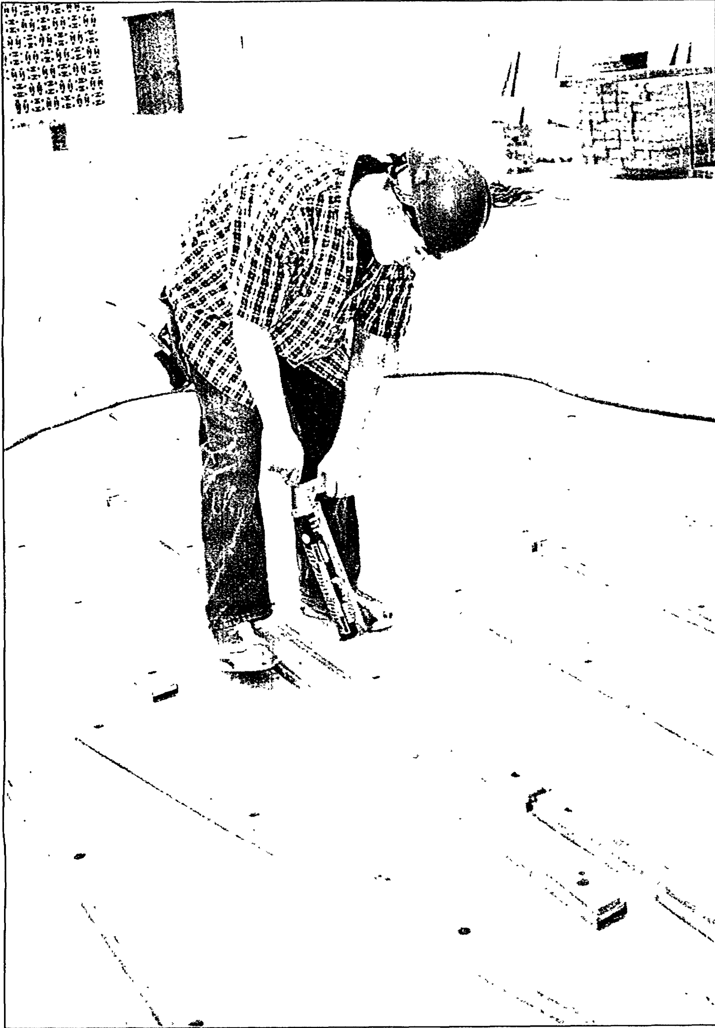
Cameron Klosner of Wixom's Specialty Floors, works on laying down the base support bridging of the wooden floor for Northville's new high school gymnasium.
