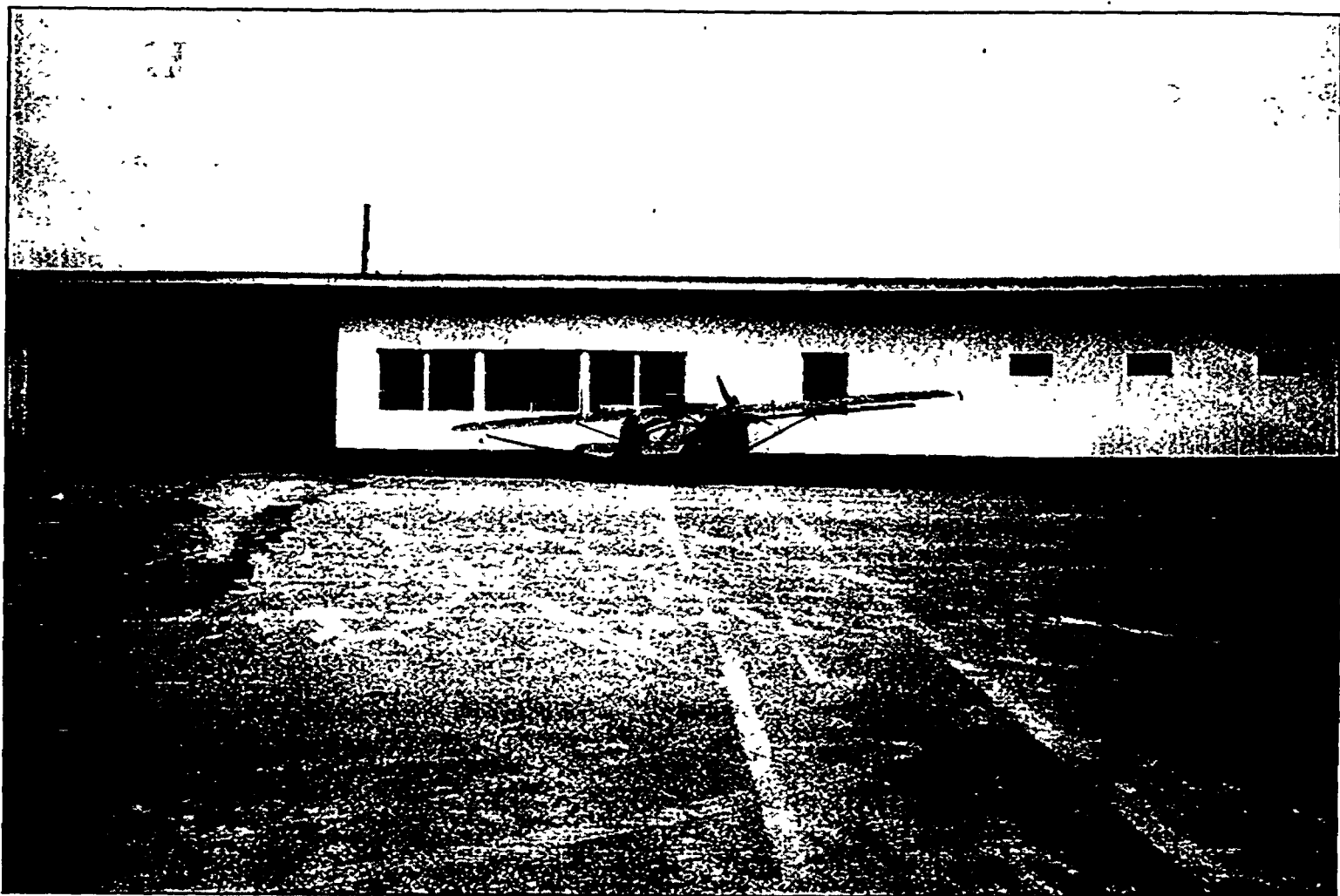
Windows were broken and cinder block walls damaged at the Northville Downs' paddock when a plane flown by a Salem man was forced to make a crash landing at the Downs. Photo courtesy HOWARD PAYNE
