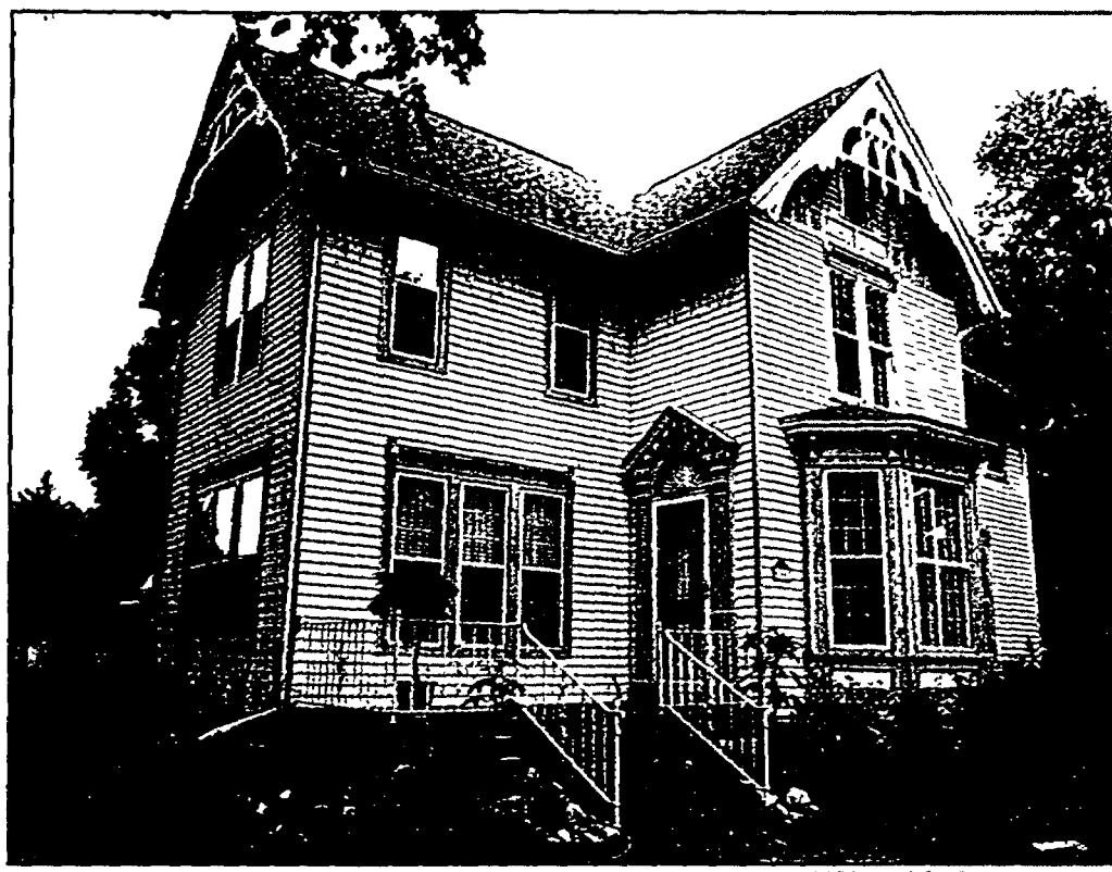
Paulson's Construction Inc. created the gingerbread trim on this house in the city of Howell from old photographs.
