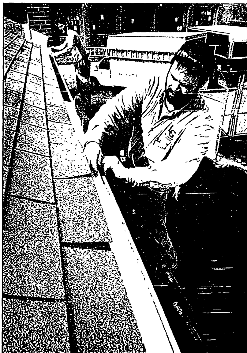
Livingston Gutter owner Dan Dancey fits new low-profile gutter helmets to existing gutters. The new material is barely visible from street level, sheds water easily and keeps gutters free of leaves and twigs.
