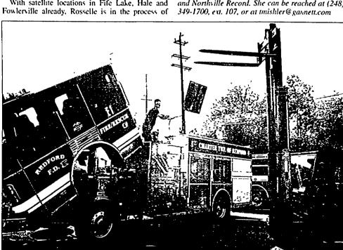
R&R Fire Truck Repair mechanic Glenn McCollum gets some help taking out a 600pound hydraulic generator from a Redford Fire Department engine.
