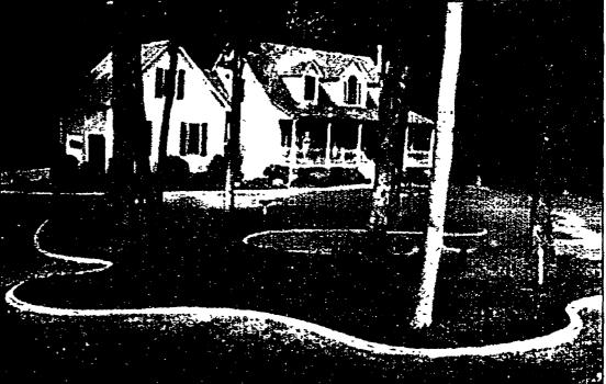
Made of mortar and fiber mesh, curbing is installed several inches into the soil to block weeds and grass from getting into landscaped areas. The bricklook pictured above shows off one of the many colors and stamped designs curbing offers. Below, curbing's flexible materials and installation process allow it to take many shapes in order to confine landscape material and stop weed invasion.
