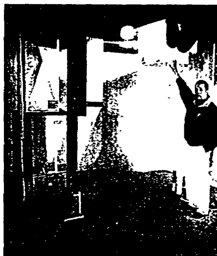
Northville's LEED Platinum Home's basement and its high-efficiency heat pump at left (note tubes at lower left that lead to its wells outside.) Doug Selby points to the home's air recirculation system, above, that helps to capture and scrub air and energy already within the home's system instead of wasting it by venting it outside.
