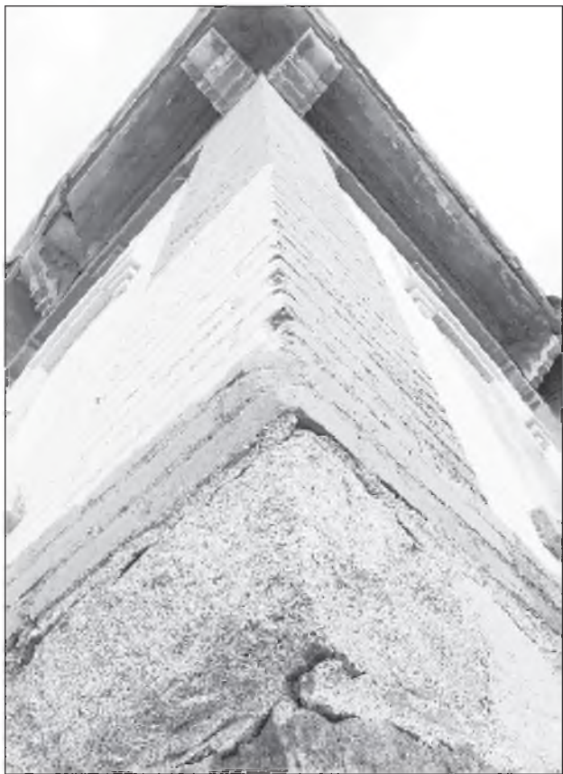
The school at Thayer's Corner shows a number of different materials used in its 1877 construction including field stone, brick and wood roof decorations.
