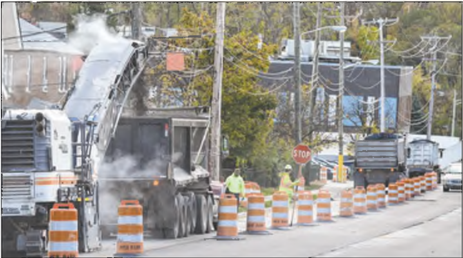
Construction crews finish up resurfacing Sheldon Road as it approaches Main Street in Northville on Oct. 23. The road has been in poor condition for years, and benefited from a new coating of asphalt. JOHN HEIDER | STAFF PHOTOGRAPHER
